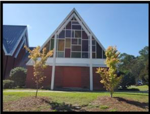
2. **Stained Glass Project:** The broken stained glass panels have been replaced. The surrounding framework, wood, and the metal archway have been painted. The 36'x2' span above the double doors has been covered in vinyl siding. The remaining items on this project are nighttime backlighting of the glass, some additional aesthetic work, an irrigation system, and landscaping.
